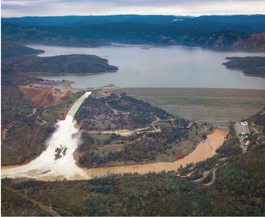
Oroville Dam’s spillways were damaged during the early February 2017 storm, ranked as an extreme landfalling atmospheric river. In addition to the damage at Oroville, multiple storms in a month that was wet statewide resulted in localized urban flooding in places as diverse as Maxwell, San Jose, and San Diego.
