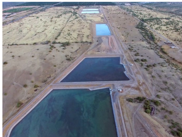
Figure MM02-5. Tonopah Desert Recharge Project Ponds (Central Arizona Project, 2021).
