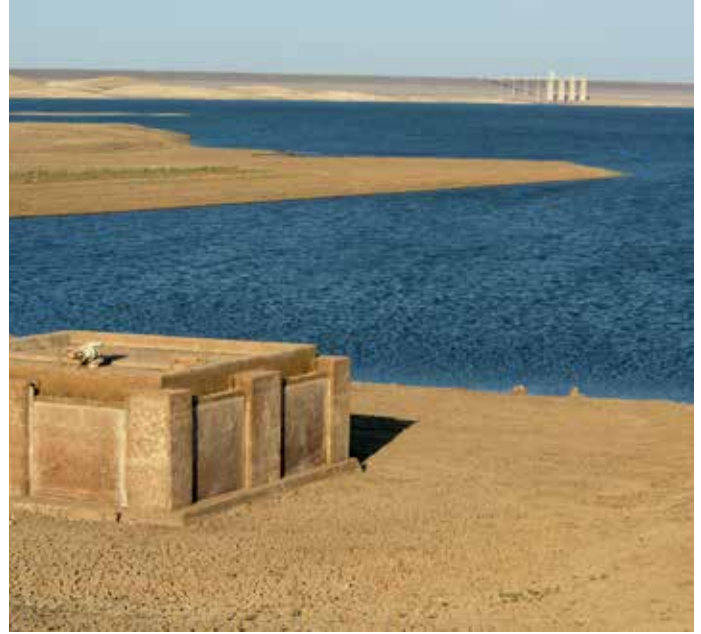
Tule elk graze on the bottom of the 2 million acre-foot state-federal San Luis Reservoir on August 24, 2016, when the reservoir was at 13 percent of its capacity. Low water levels exposed the upper intake structure for San Felipe Division of the Central Valley Project, which supplies water to Santa Clara Valley Water District and to San Benito County Water District. The intake has also been exposed in other drought years, such as 1991 and 2008. Low water levels in the reservoir in late summer lead to a problem known as “low point” for the San Felipe Division contractors, when reduced reservoir volume and warm temperatures contribute to growth of a thick layer of algae. The algae create drinking water taste and odor problems for urban water users, and clog drip irrigation systems for agricultural water users.
