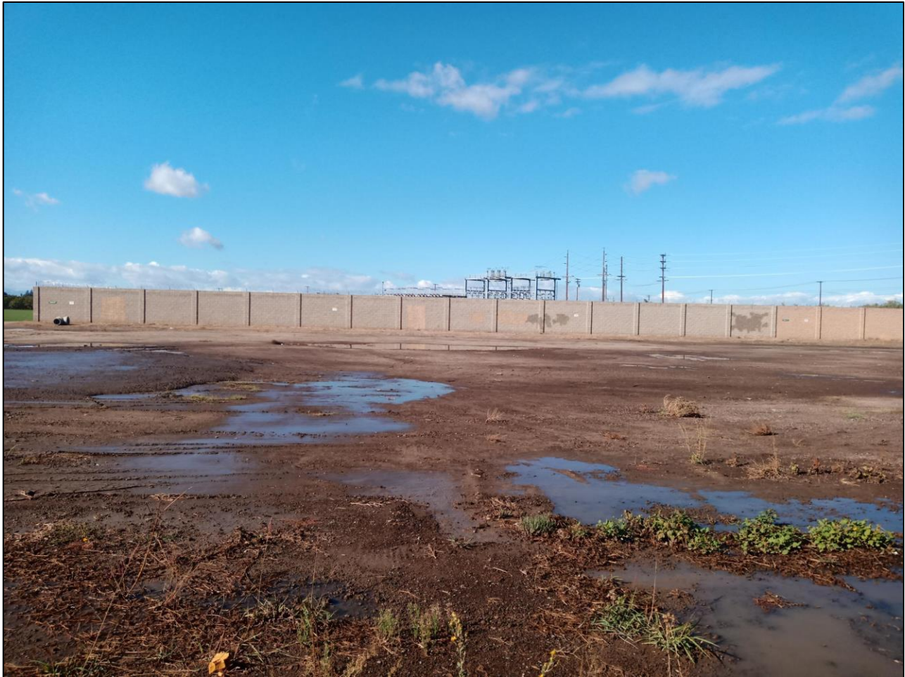
Figure 3. Overview of Proposed Generator Installation Area. View to the east.
