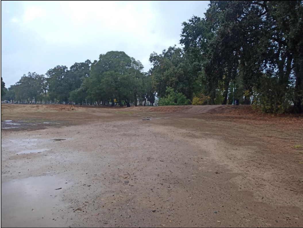
Figure 4. Overview of Proposed Generator Installation Area. View to the north.
