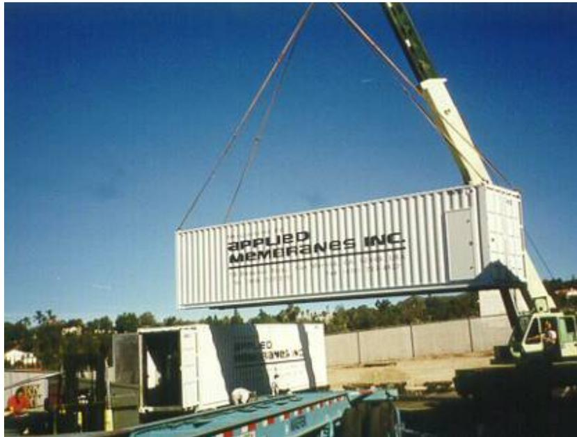
Crane Lifted Containerized Mobile Desalination Unit
