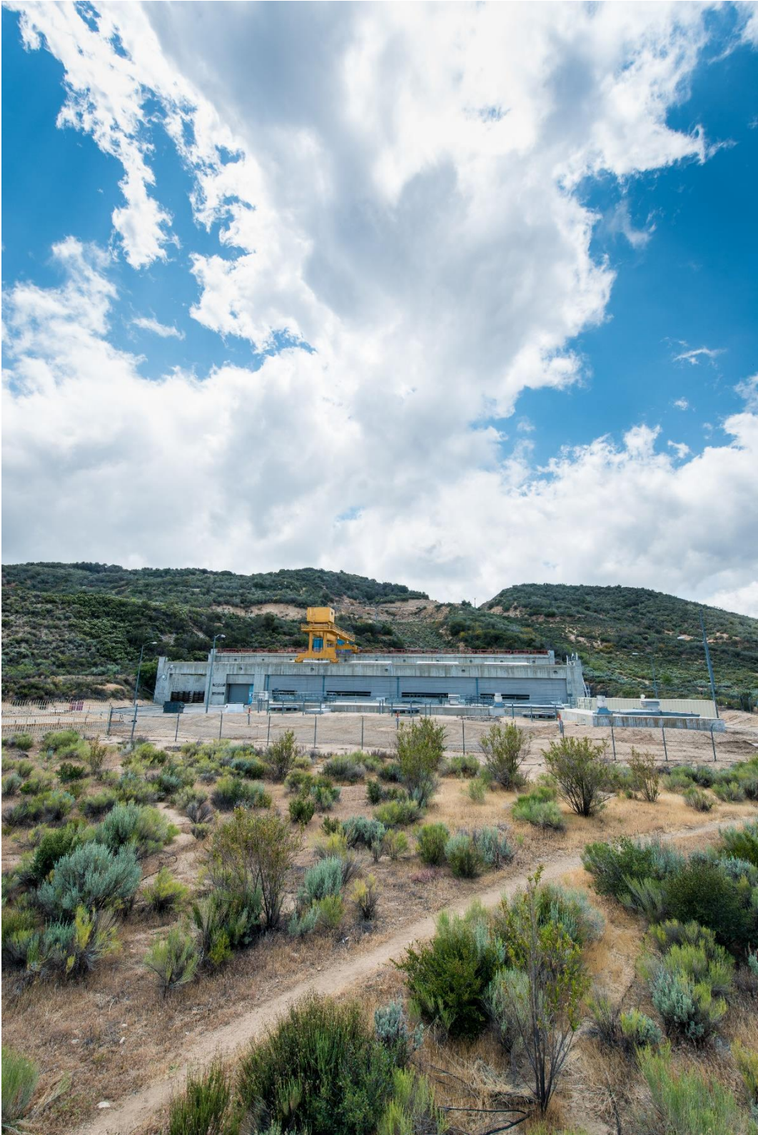
Photo 11 Mojave Siphon Powerplant
