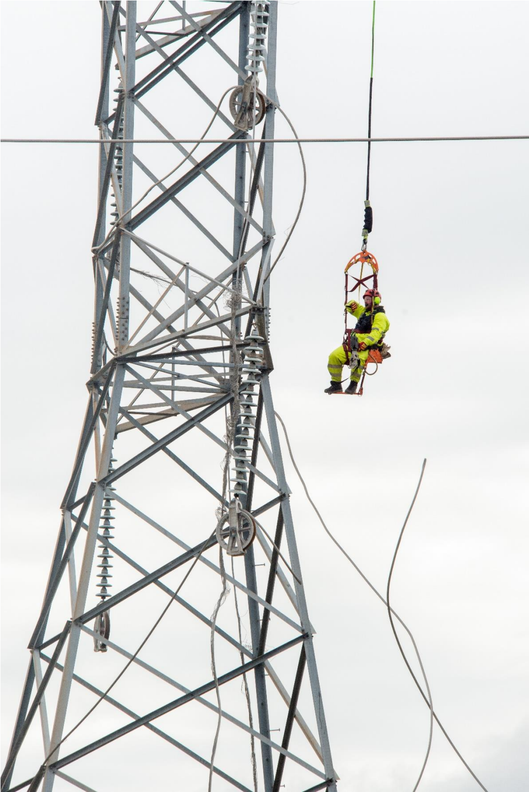
Photo 17 Power Line Worker in Oroville
