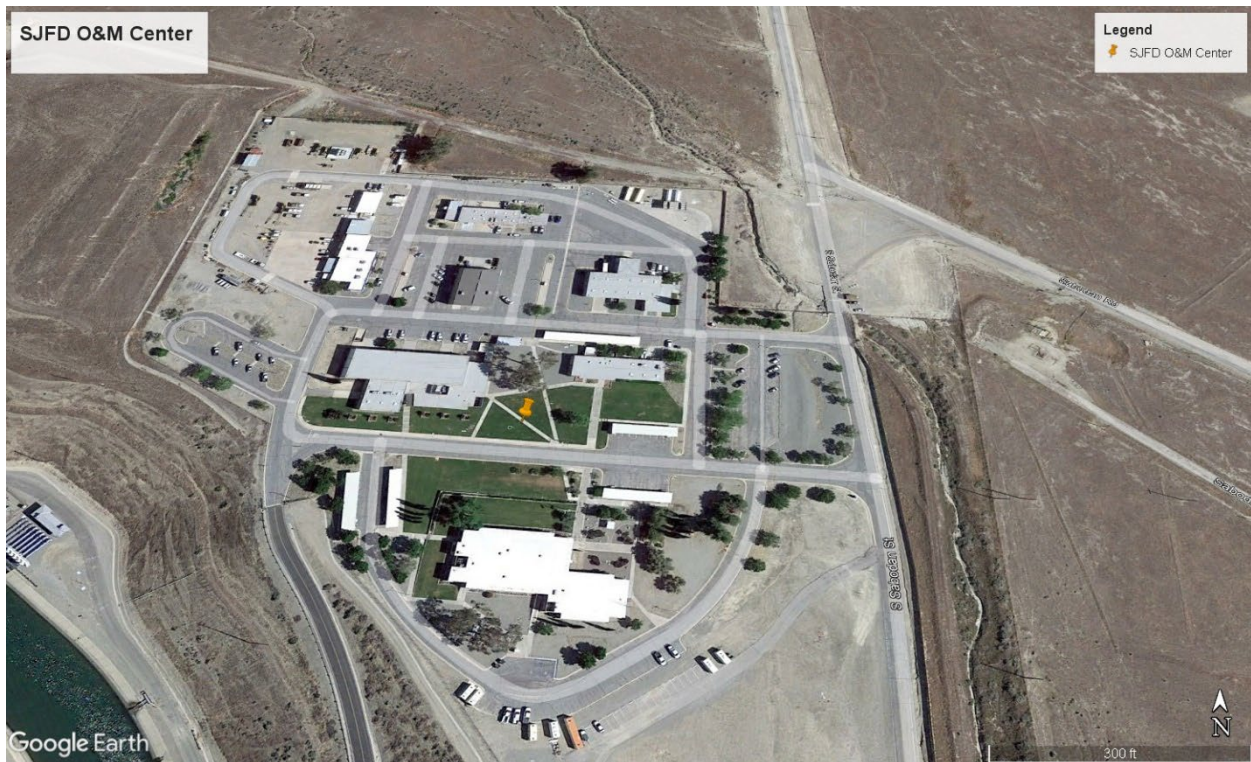
Figure 2-3: SJFD O&M Center
