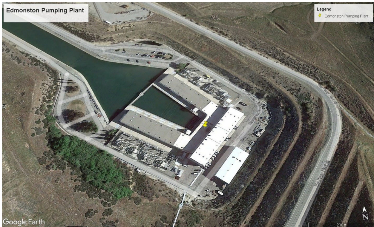
Figure 2-6: Edmonston Pumping Plant
